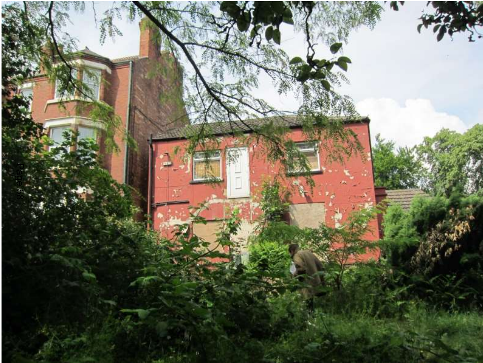
Existing building – rear elevation
